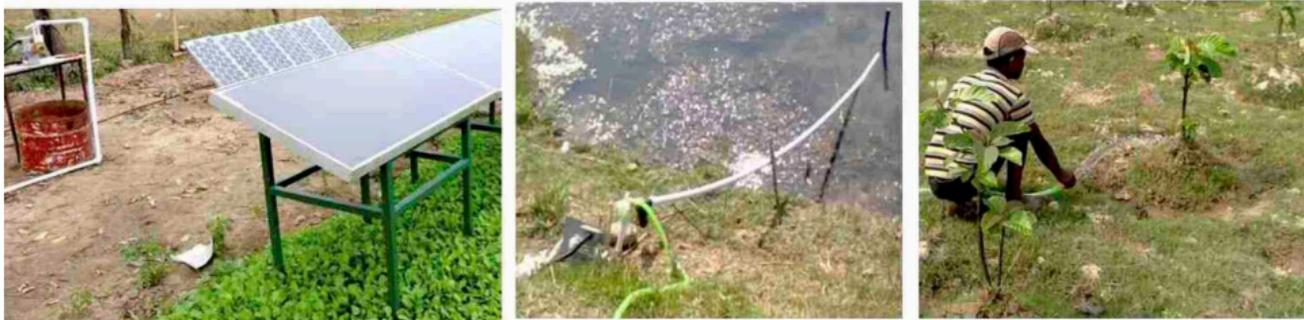
**Irrigation water service provided by micro-grid driven pump or mobile units with solar PV or battery)**
